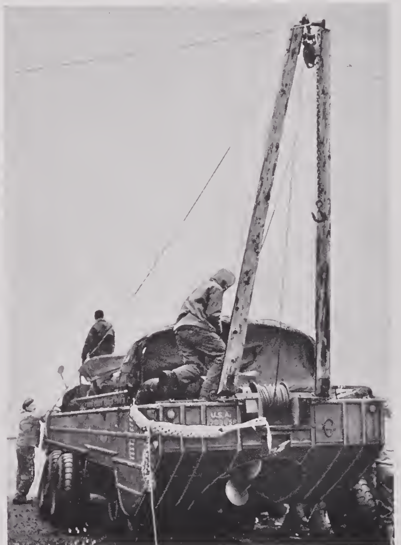
FIGURE 55. Emergency A-frame improvised from cedar timbers for demonstration at Provincetown, Massachusetts.
